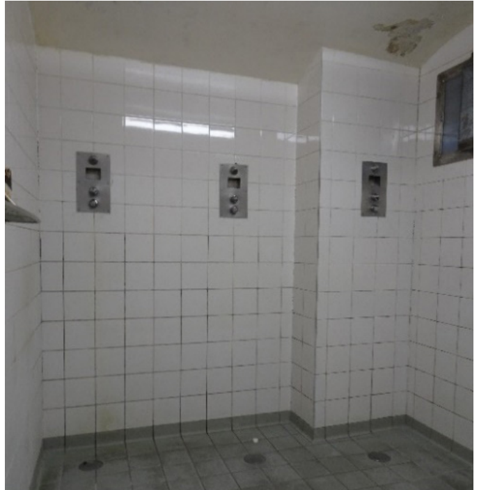
Area 1 communal shower block (January 2025)
