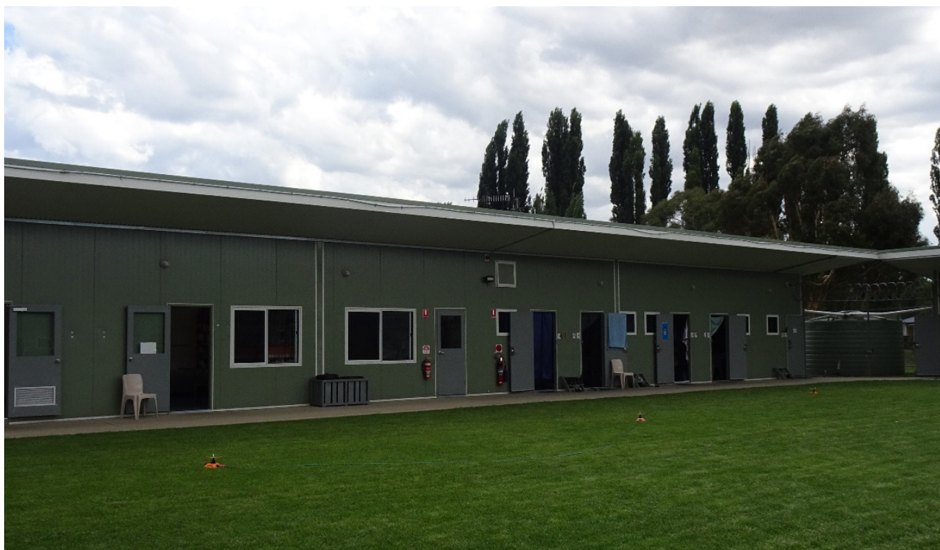
Area 2 yard and accommodation building
