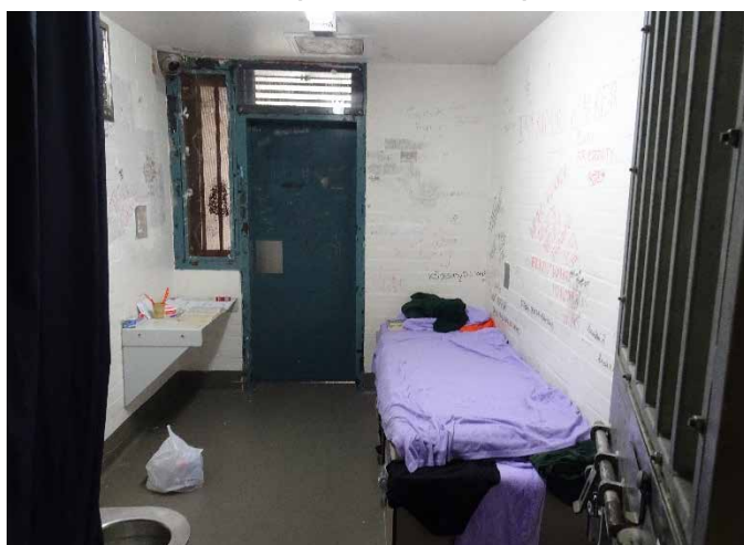
Induction unit cell (unrefurbished)
