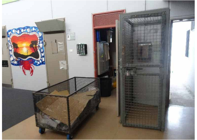
Telephone in cage
