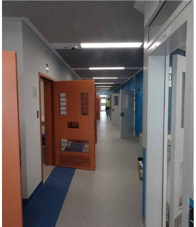
Corridor between cells in the new MPU
