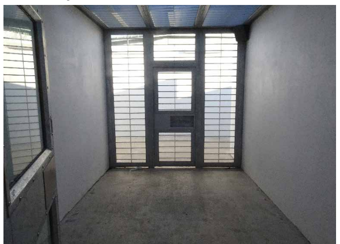
Exercise yard at rear of MPU cell
