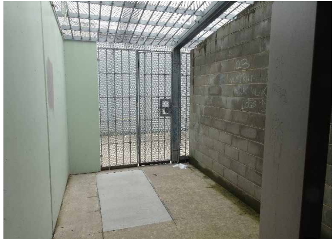
Exercise yard connected at rear of cell
