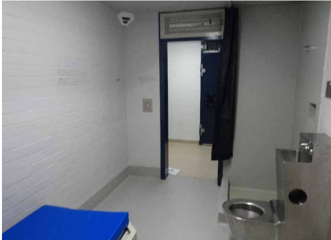
Induction unit cell with CCTV directly facing toilet
