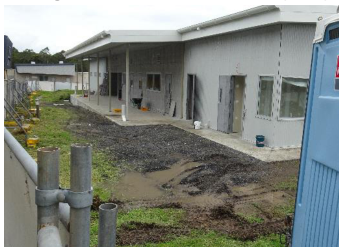
Building in Sector 1- under construction (2023)
