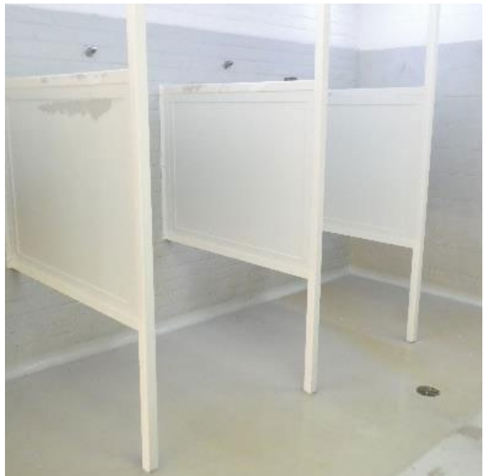
2024 refurbishment of shower block
