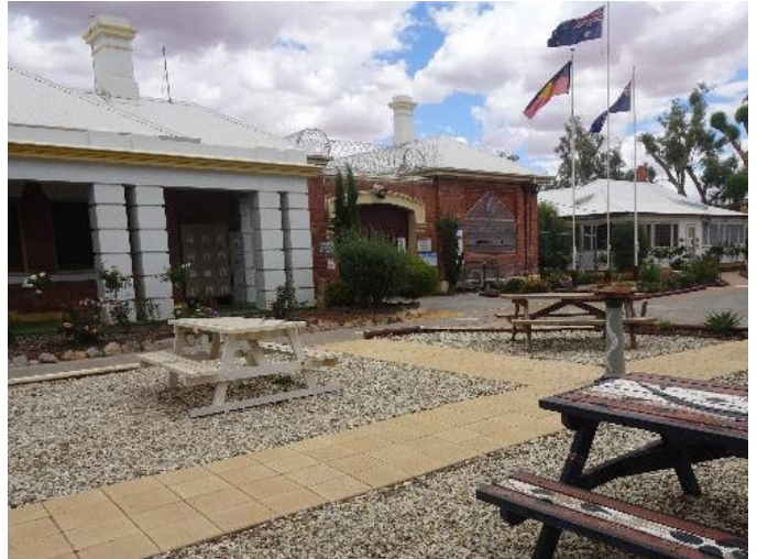
Flagpoles at Broken Hill CC
