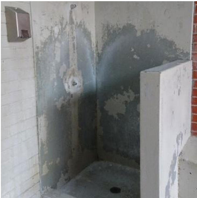
Shower block in rear holding yard
