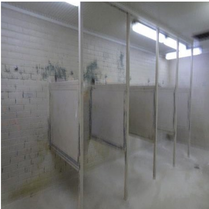
Shower block in the long yard
