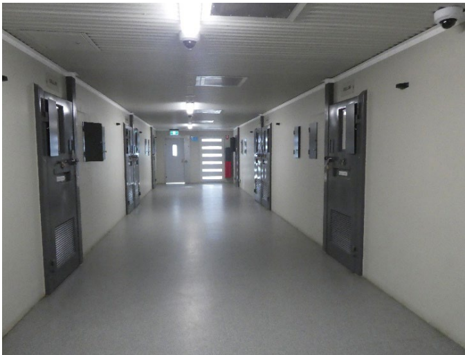
Cell doors and corridor, women's unit (FTU)
