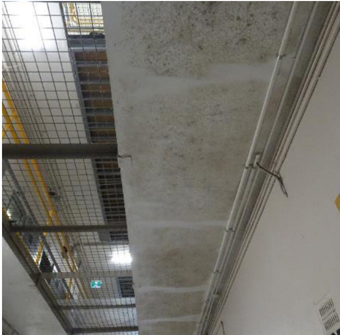
Mould on 13-wing ground landing ceiling, February 2024
