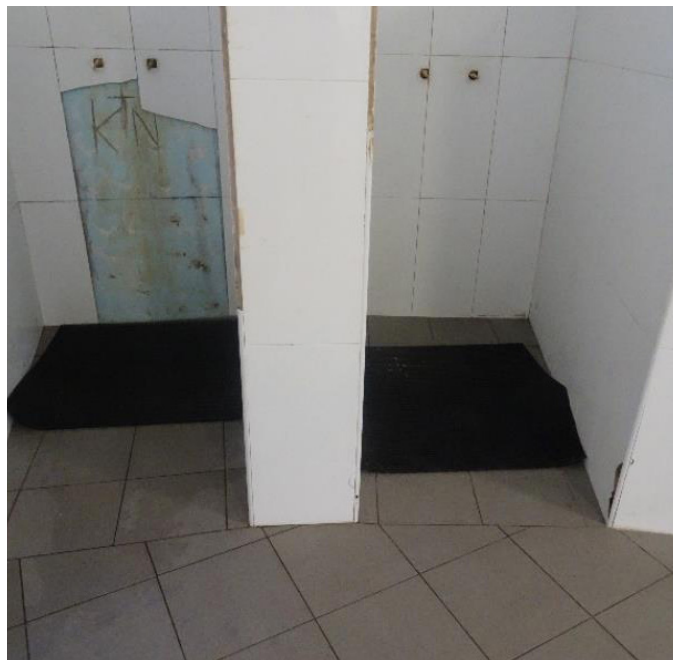
MSPC 1, 7-wing showers with broken tiles and slip hazards, May 2024
