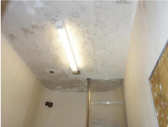
Mouldy and damaged cell ceilings in 5-wing, May 2024
