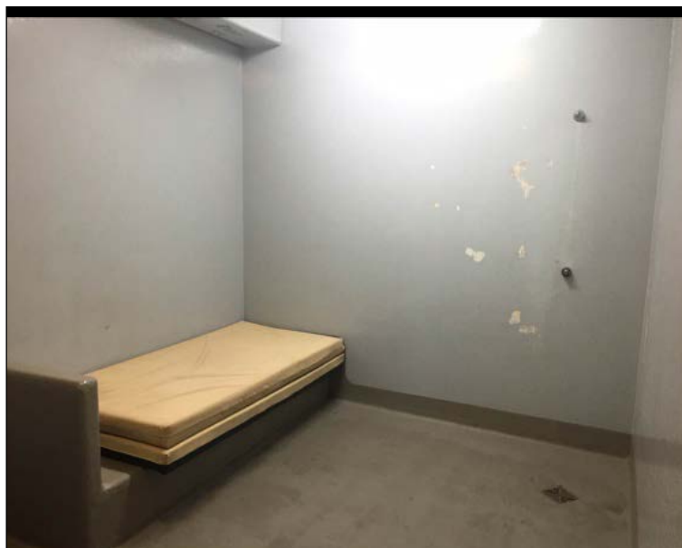
Shower in cell with no barrier
