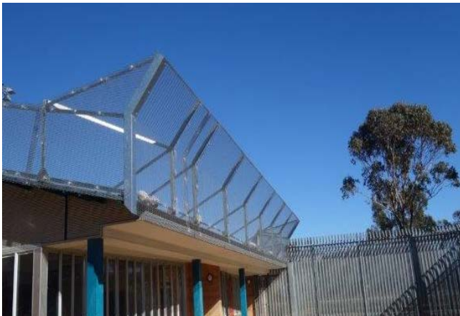
Anti-climb structure at Orana YJC
